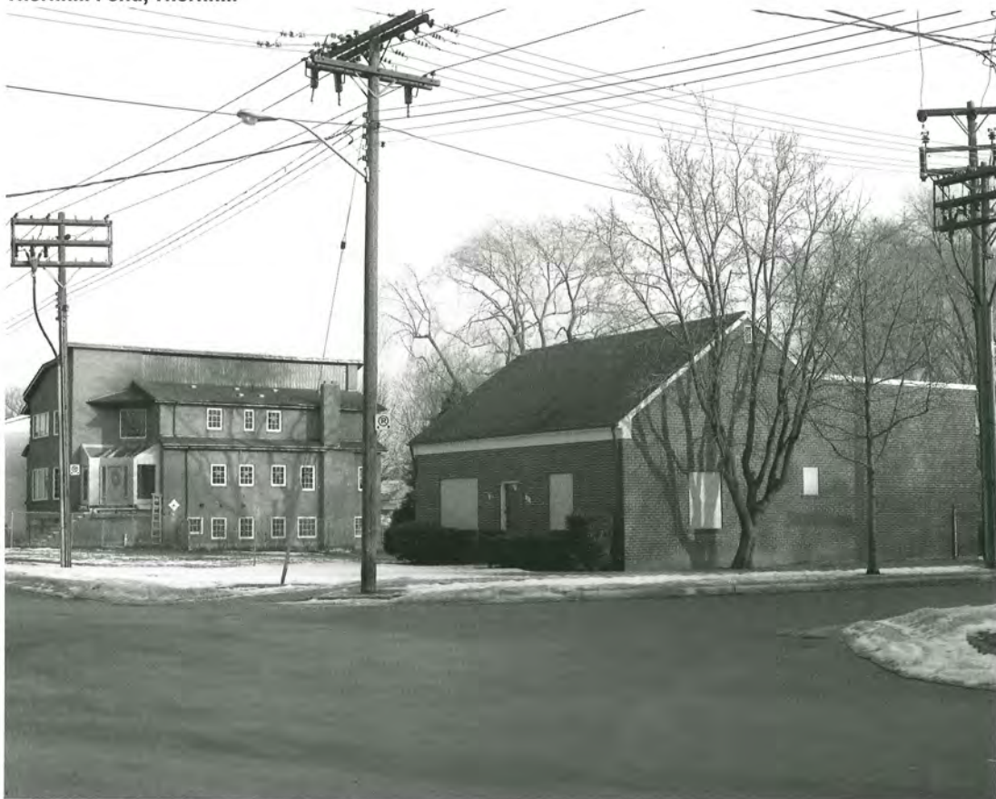
83 – 85 Pemberton Avenue, North York
